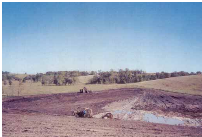
This soil erosion structure (pond) was constructed in cooperation with a neighboring landowner to control a gully in a boundary fence.
